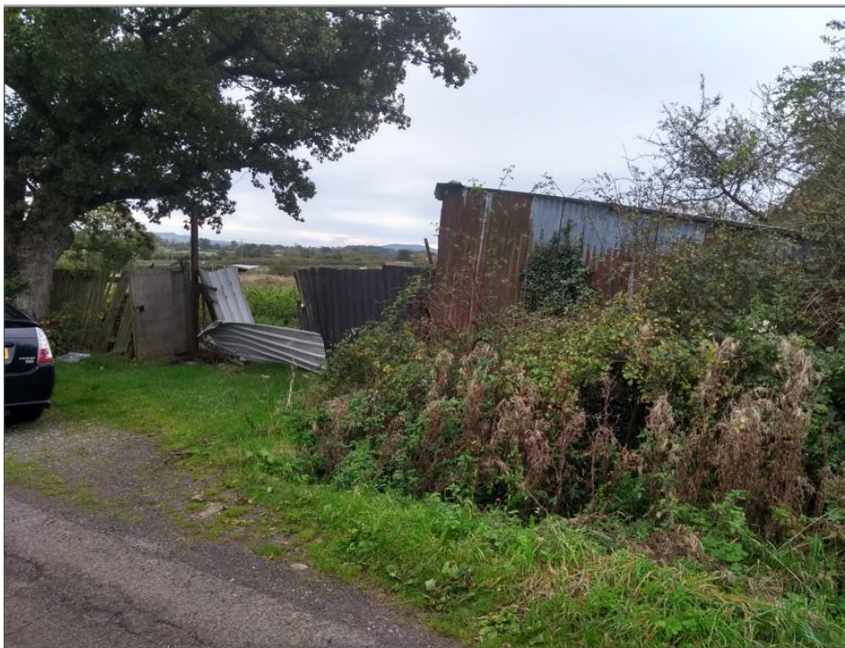
View of existing access from highway
